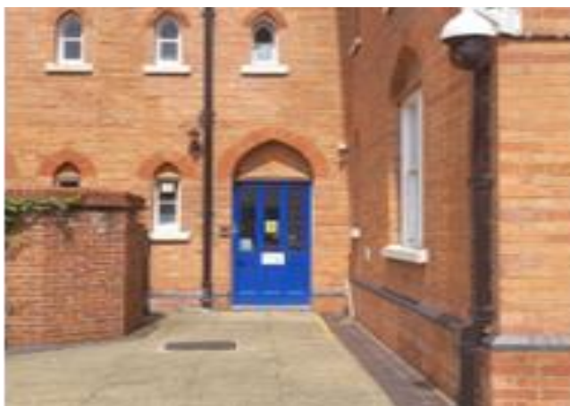
Car Park Entrance (rear of building)
